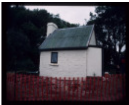
LIMESTONE COTTAGE EXCAVATION
