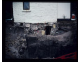
LIMESTONE COTTAGE EXCAVATION
