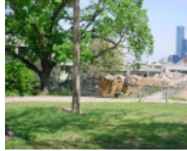
h02009 js 10 nov 2003 southern elm during demolition
