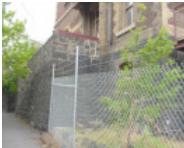
h02009 mornington wall 2 nov 2003
