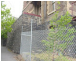
h02009 mornington wall 2 nov 2003
