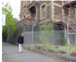
h02009 mornington wall 1 nov 2003
