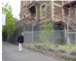
h02009 mornington wall 1 nov 2003
