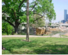
h02009 js 10 nov 2003 southern elm during demolition
