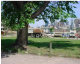
h02009 js demolition 10 nov 2003
