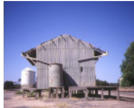
murrayville railway station mckenzie street murrayville goods shed side view apr1995
