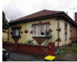
Richmond Charlotte Street 13-15.JPG
