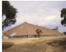
murtoa grain store wimmera hwy murtoa site view
