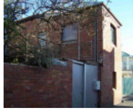
Carlton North Amess Street 261rear v3.JPG
