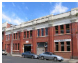
Rear of 7 Stanley Street
