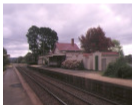
new gisborne railway station compelx station road trackside view apr1995
