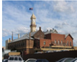
Rear of Town Hall (from Gleadell Street)
