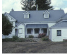
woolamai house cleeland road woolamai waters phillip island rear view
