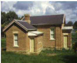
newstead court house conrobert street newstead side view sep 97
