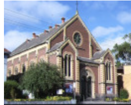
1 baptist church aberdeen street newtown front view
