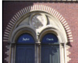
baptist church aberdeen street newtown detail entrance
