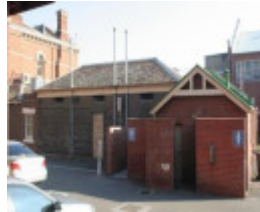
Richmond Police Station - bluestone police cells at the rear
