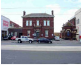
Richmond Police Station
