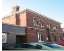
Richmond Police Station
