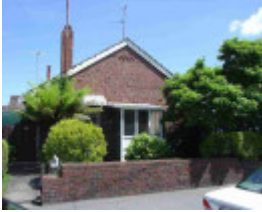
burnley bridge road burnley bridge road 640
