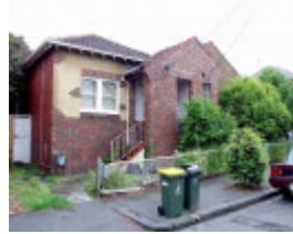
Richmond Charlotte Street 7- 9.JPG
