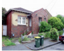
Richmond Charlotte Street 7- 9.JPG
