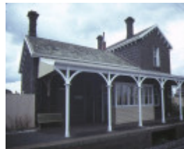
1 bannockburn railway station rear elevation aug1984
