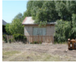
BANNOCKBURN RAILWAY STATION SOHE 2008
