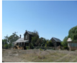
BANNOCKBURN RAILWAY STATION SOHE 2008
