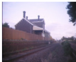
bannockburn railway station side view apr1995
