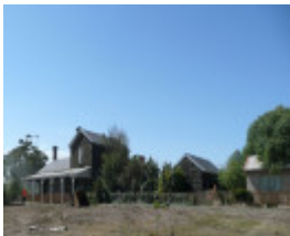
BANNOCKBURN RAILWAY STATION SOHE 2008
