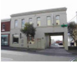
collingwood johnston street collingwood johnston street 40
