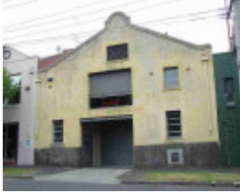
richmond clifton street richmond clifton street 9a
