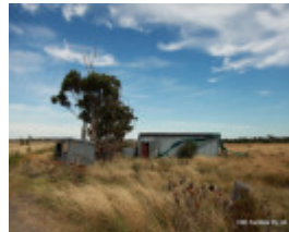
Clean-up re. asbestos 2012
