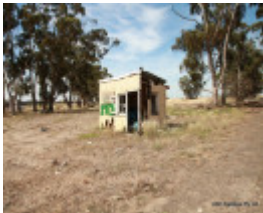
Clean-up re. asbestos 2012
