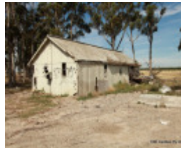
Clean-up re. asbestos 2012
