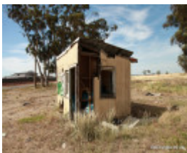
Clean-up re. asbestos 2012
