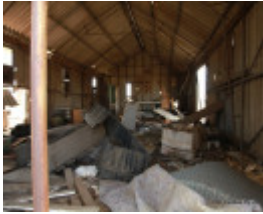
Clean-up re. asbestos 2012
