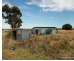
Clean-up re. asbestos 2012
