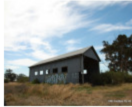
Clean-up re. asbestos 2012
