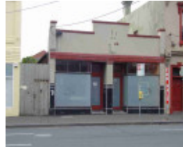
Collingwood Johnston Street 160-162.JPG
