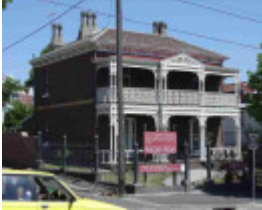
richmond church street richmond church street 300
