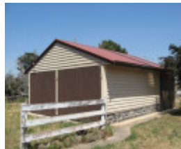
Clonard homestead complex_garage
