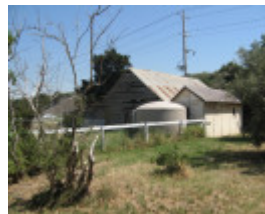
Clonard_milking/shearing shed and milking machine shed
