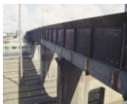
north melbourne railway station railway place north melbourne footbridge sep1998
