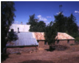
the hermitage murray valley hwy barnawartha outbuildings
