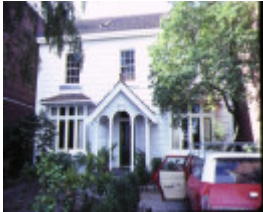
1 456 victoria street nth melb front view
