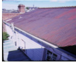
456 victoria street nth melb roof back
