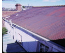
456 victoria street nth melb roof back
