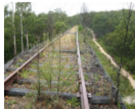
Top of bridge, Jan 2008.
