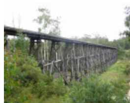
General view of bridge, Jan 2008.
