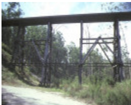
rail bridge nowa nowa trestle detail feb1985
