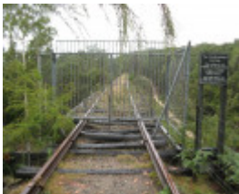
Top of bridge, Jan 2008.
