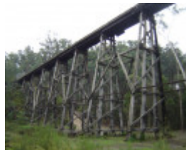
General view of bridge, May 2007.
