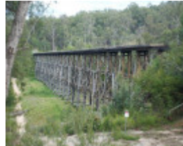
RAIL BRIDGE SOHE 2008
