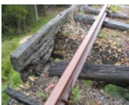
Rail and sleepers detail, Jan 2008.
