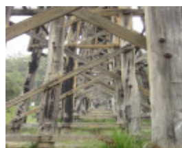
Bridge structure, May 2007.
