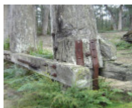
Bridge piles detail, May 2007.
