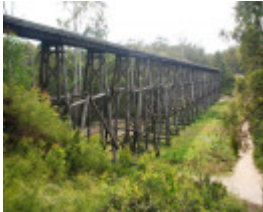
RAIL BRIDGE SOHE 2008
