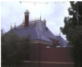
numurkah court house melville street numurkah side view roof detail nov1984
