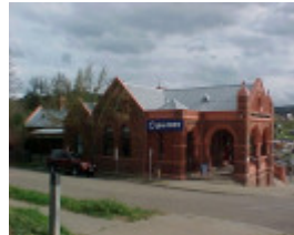
former omeo post office corner view oct1999
