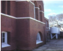
former omeo post office side wall jul1980
