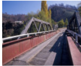
h00917 hinnomunjie bridge over mitta mitta river omeo from omeo end she project 2003
