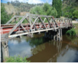
HINNOMUNJIE BRIDGE SOHE 2008
