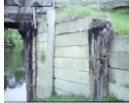
hinnomunjie bridge omeo river bank supports
