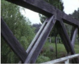
hinnomunjie bridge omeo detail of wooden beams
