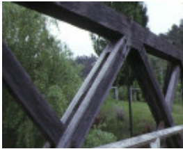
hinnomunjie bridge omeo detail of wooden beams
