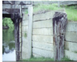
hinnomunjie bridge omeo river bank supports
