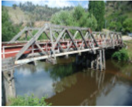
HINNOMUNJIE BRIDGE SOHE 2008
