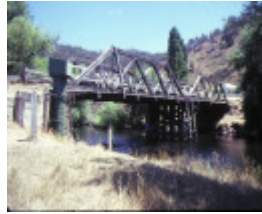
1 hinnomunjie bridge omeo side view feb1985
