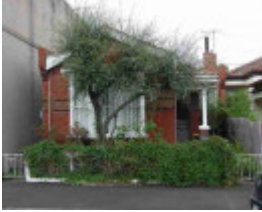
princes hill holtom street princes hill holtom street 24
