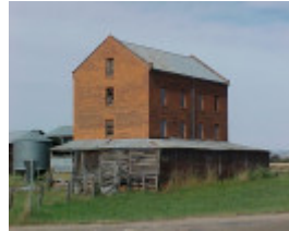
1 former flour mill oxley nov99
