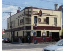
Bridge Road 470.JPG
