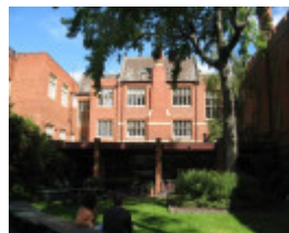
JCH rear (east side) of main wing and courtyard addition
