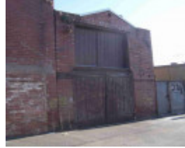
Rear of 28 McIlwraith Street.JPG
