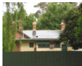
view from rear yard with flat roofed infill extension
