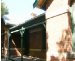
FORMER POLICE STATION COMPLEX SOHE 2008
