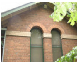
segmental arched window pair to facade
