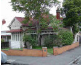
richmond malleson street richmond malleson street 2
