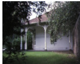
nocklofty royal parade parkville verandah dec1978
