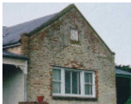
laurence park homestead buchter road batesford front window detail publication
