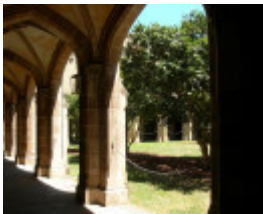
LAW SCHOOL BUILDING AND OLD QUADRANGLE SOHE 2008
