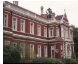
1888 building university of Melbourne parkville side elevation
