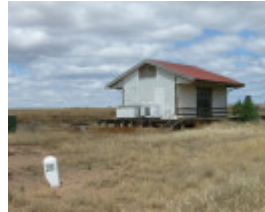
PATCHEWOLLOCK RAILWAY STATION COMPLEX SOHE 2008
