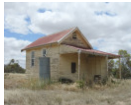
PATCHEWOLLOCK RAILWAY STATION COMPLEX SOHE 2008
