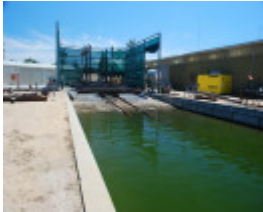
SLIP AND WINCH SHED SOHE 2008
