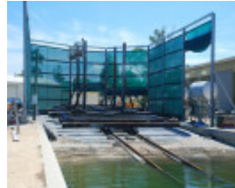
SLIP AND WINCH SHED SOHE 2008
