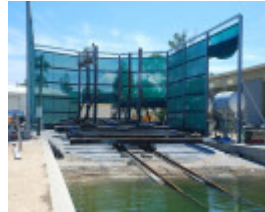
SLIP AND WINCH SHED SOHE 2008
