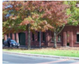
Cable Tram Engine House
