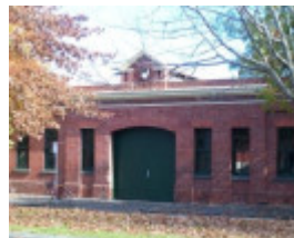
Cable Tram Engine House
