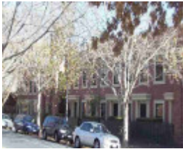
Cable Tram Engine House
