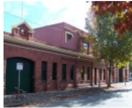
Cable Tram Engine House
