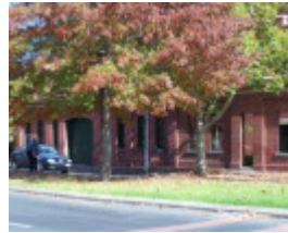
Cable Tram Engine House
