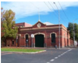
Cable Tram Engine House
