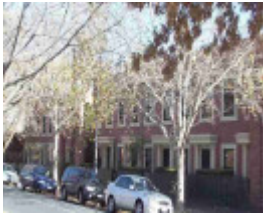
Cable Tram Engine House
