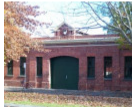
Cable Tram Engine House
