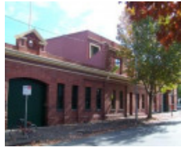
Cable Tram Engine House
