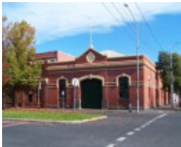
Cable Tram Engine House
