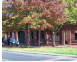
Cable Tram Engine House
