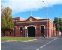
Cable Tram Engine House
