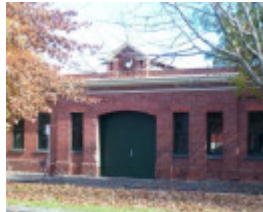
Cable Tram Engine House
