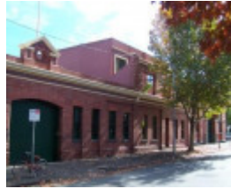
Cable Tram Engine House
