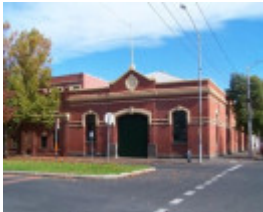
Cable Tram Engine House
