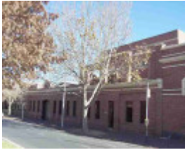
Cable Tram Engine House - 1023 Rathdowne
