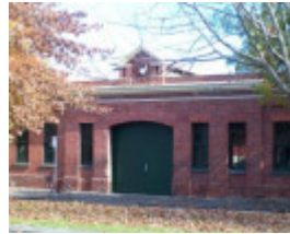
Cable Tram Engine House
