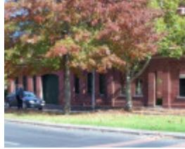
Cable Tram Engine House
