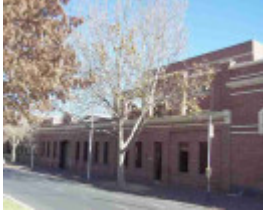
Cable Tram Engine House - 1023 Rathdowne
