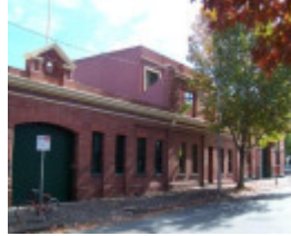
Cable Tram Engine House
