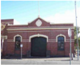
Cable Tram Engine House - 1025 Rathdowne
