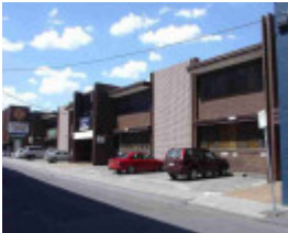
richmond wangaratta street richmond wangaratta street 31-43
