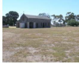
POINT COOK HOMESTEAD AND STABLES SOHE 2008
