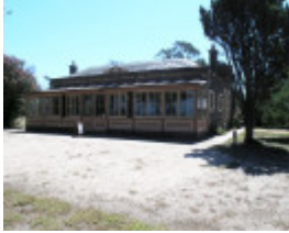
POINT COOK HOMESTEAD AND STABLES SOHE 2008
