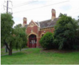
princes hill solly avenue princes hill solly avenue 20
